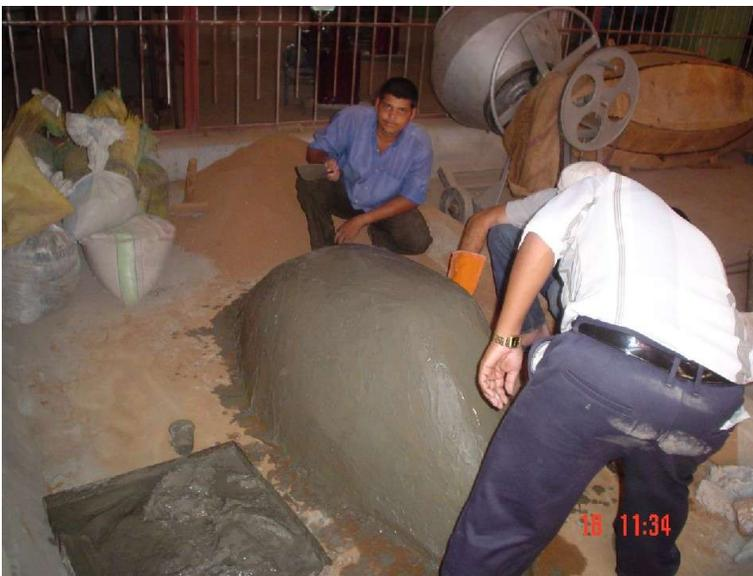
Figure 6. Model ferro-cement boat being finished.
